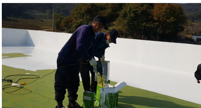
Installing a cool roof for climate crisis safe villages (Sandong-ri, Seochon-gun) (before installation: 24.1°C > after installation: 14.1°C)
